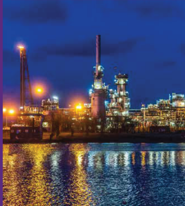
The St Fergus gas terminal. Credit: North Sea Midstream Partners (NSMP) Limited
